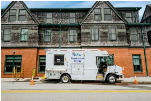
RIE crews complete underground electric upgrades in Newport
