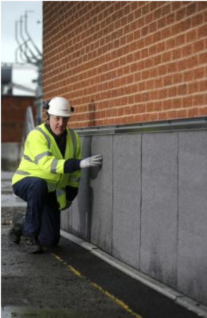
WPD's Andrew Mason checking one of the new flood walls built to protect electrical equipment from flood water.
