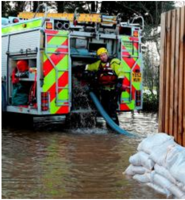
WPD's Mark Picken uses an emergency response vehicle to pump water out of a substation.
