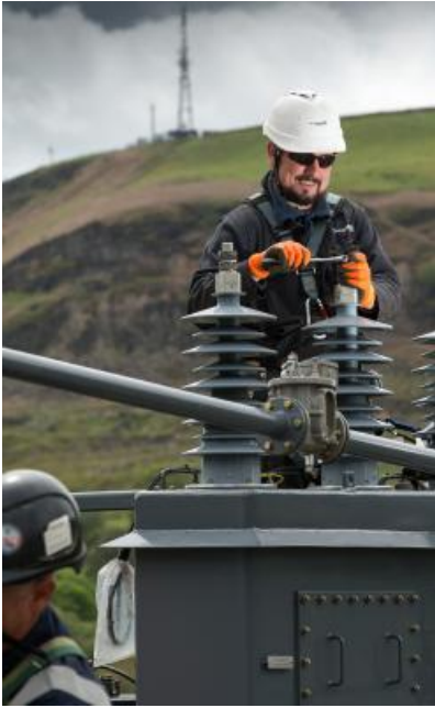
WPD Fitter Simon Bubb installing the new transformer.
