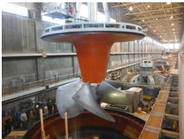
A new, state-of-the-art turbine is lowered into place during the modernization effort at the Ohio Falls hydro station.
