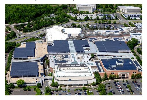
The Mall at Short Hills in New Jersey now features a 3.49 MW solar rooftop and parking deck system developed by Safari Energy.
